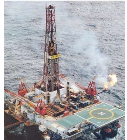
Typical Pemex Cantarell platform
